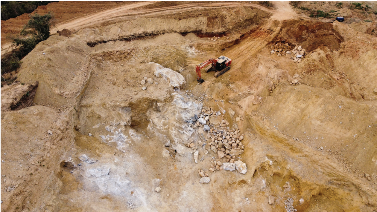
Fig 01: Mushroom technologies ltd gypsum mine site
